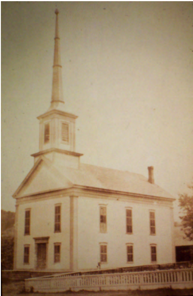
9. Baptist Church with steeple
