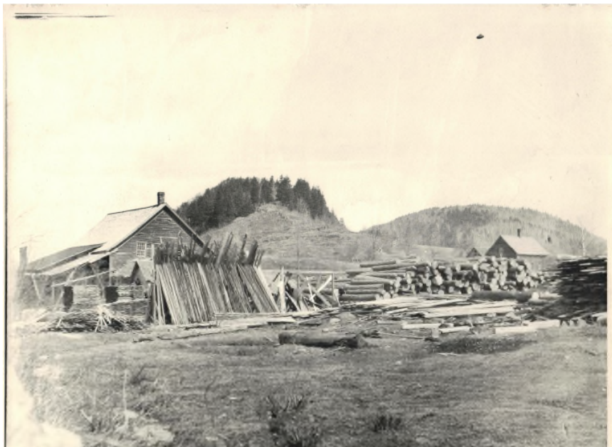
Oscar Baldwin's saw mill and cheese box factory on the pond above Starksboro village. Note the cleared hill behind the mill.
