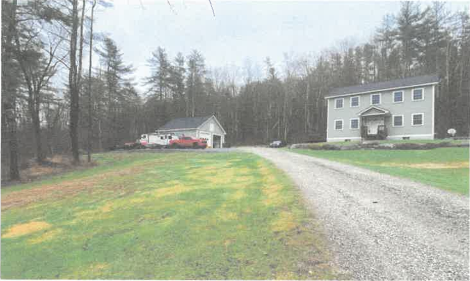
Facing N/E (below)
