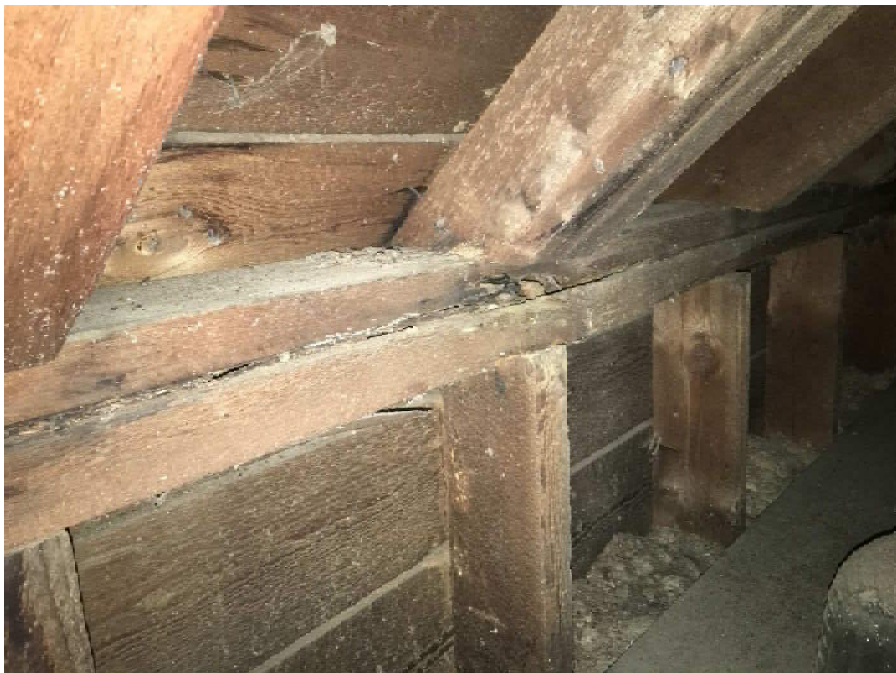
PHOTO 7: ROT AT TOP PLATE
