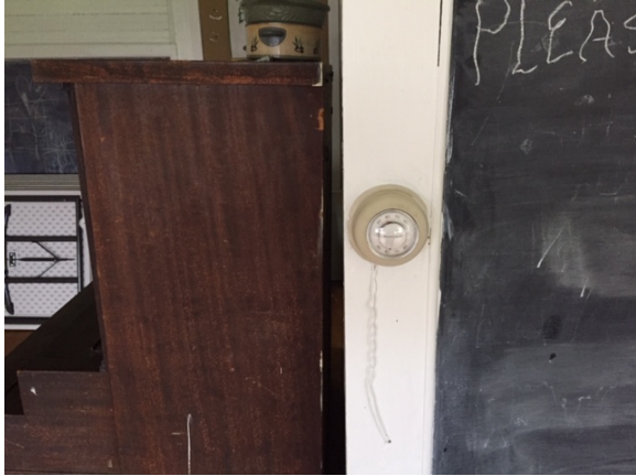
Photo #1 CPAI Area #02 – Mercury Thermostat
